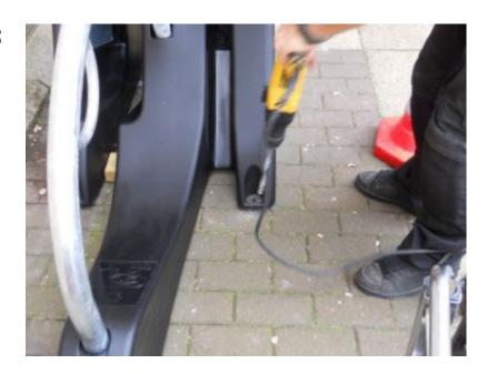
STEP 3 - AFTER DRILLING HOLES, CLEAN/BLOW OUT THE DRILLED AREA TO REMOVE ANY DEBRIS
