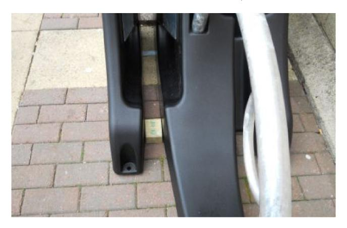
STEP 2 - USING THE SECURING POINTS AS REFERENCE, DRILL HOLES INTO THE AREA TO BE SECURED.
