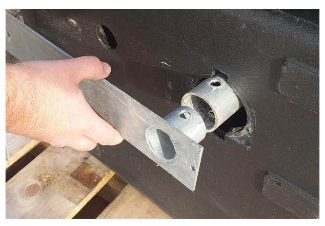
STEP 5 - Drill plates into position using 5MM (10g) x 25MM wood screws, ensuring that the holes in the metalwork line up with the holes in the streetpod.
